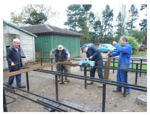
The photo above shows some of the team in action during a working session. The guys are bending rebar into hoops using Gerry's rail-bender machine. These hoops will form part of the reinforced steel work going over Ted's arched brickwork on the GLR tunnel.
